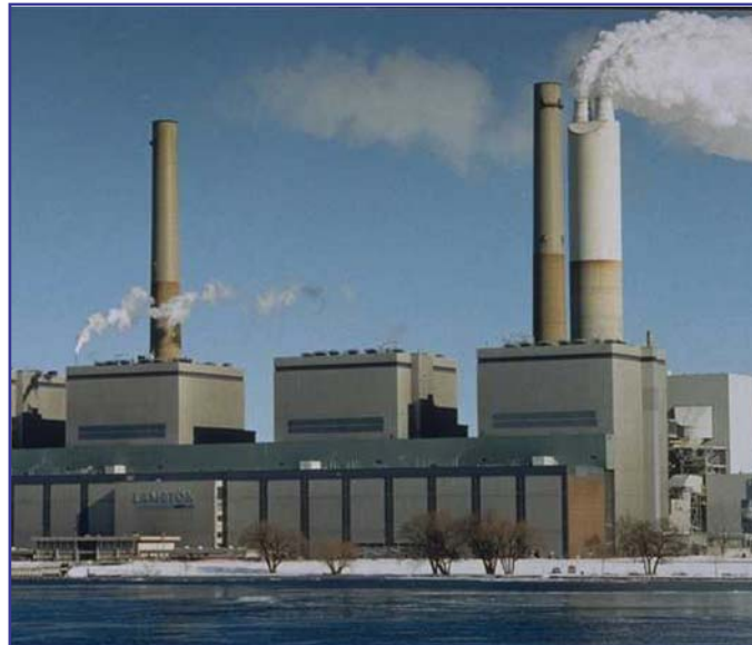
Lambton GS units lean, clean generating machines—Energy Probe
