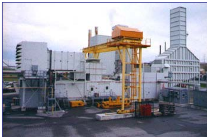
Calpine is part-owner of this 50MW co-generation facility in Whitby
