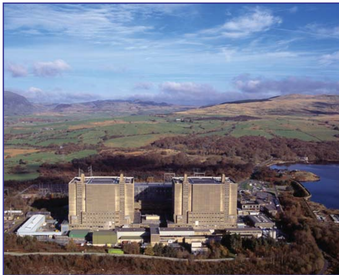
Trawsfynydd Nuclear Power Plant, Wales, UK
