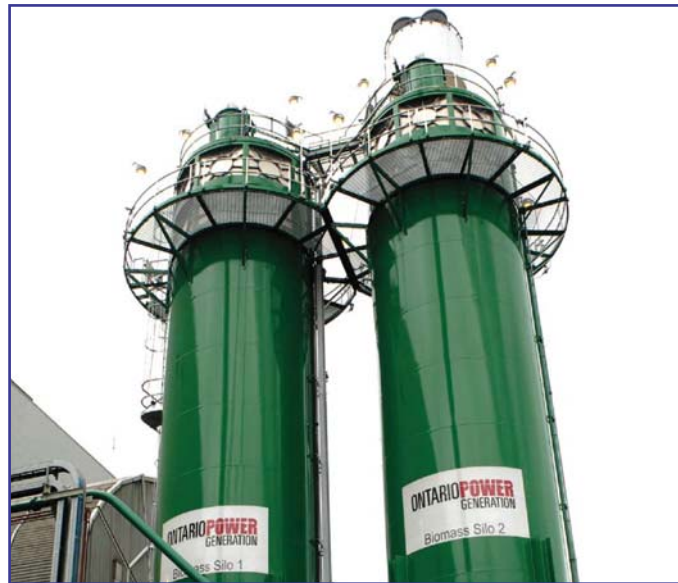
Biomass towers at OPG's Nanticoke GS
